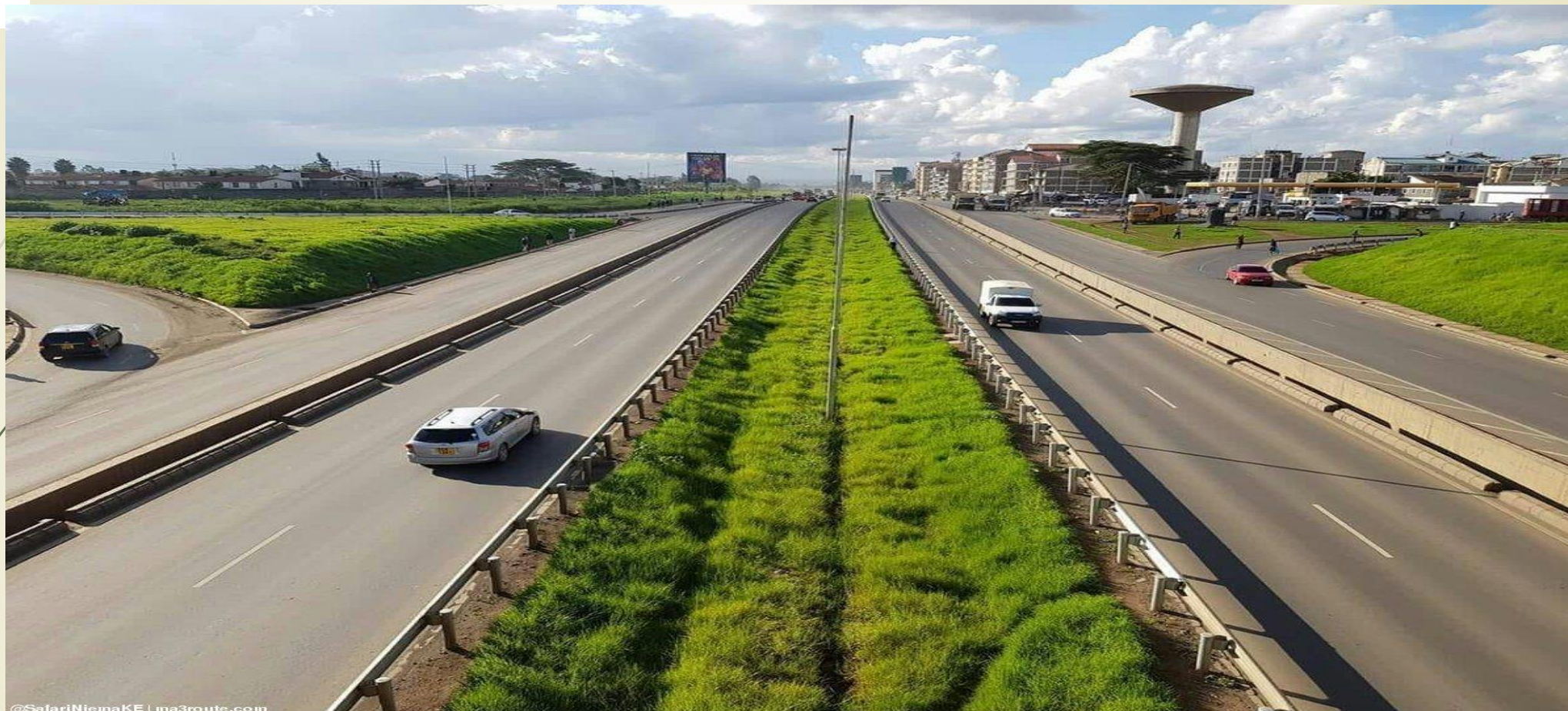
Section of Outer Ring Road showing space left out for future BRT lanes
